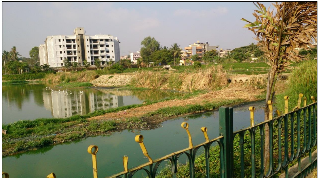
Other side of the barrier (gutters)-
