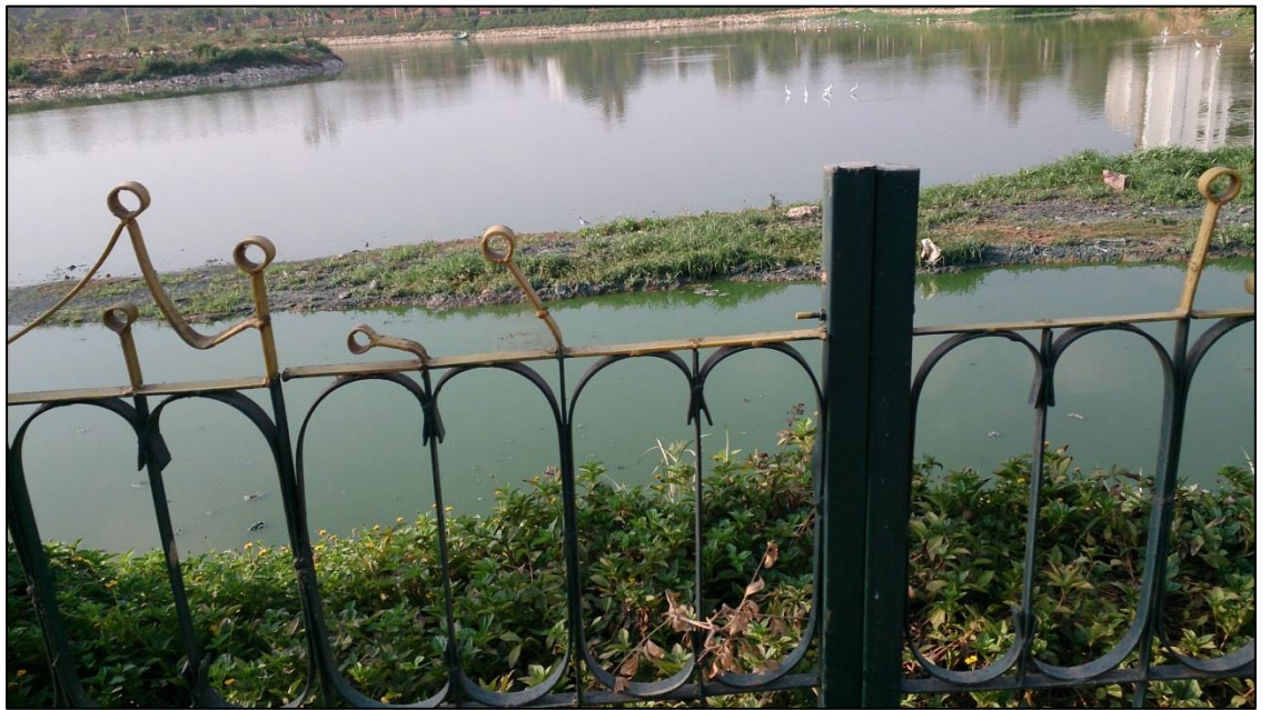
Barrier bund made to separate untreated sewage inlet from the lake-
